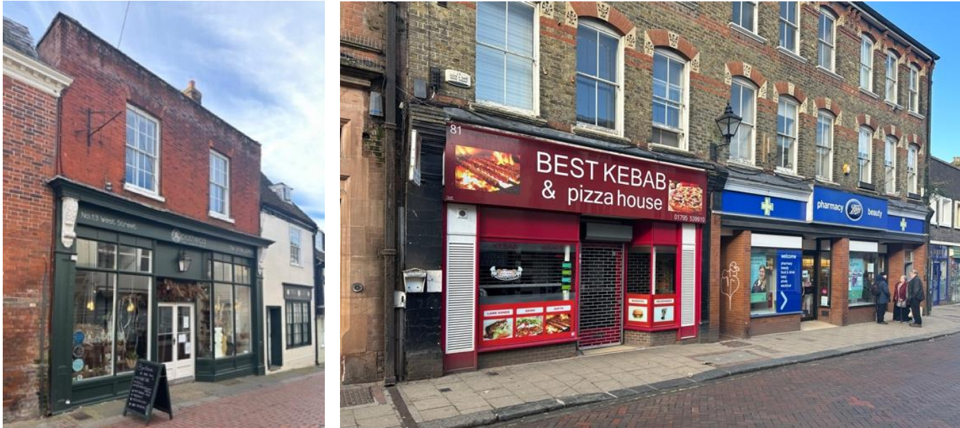
Signage: The example on the left has a sensitively designed fascia sign. The examples on the right are much more obtrusive.
